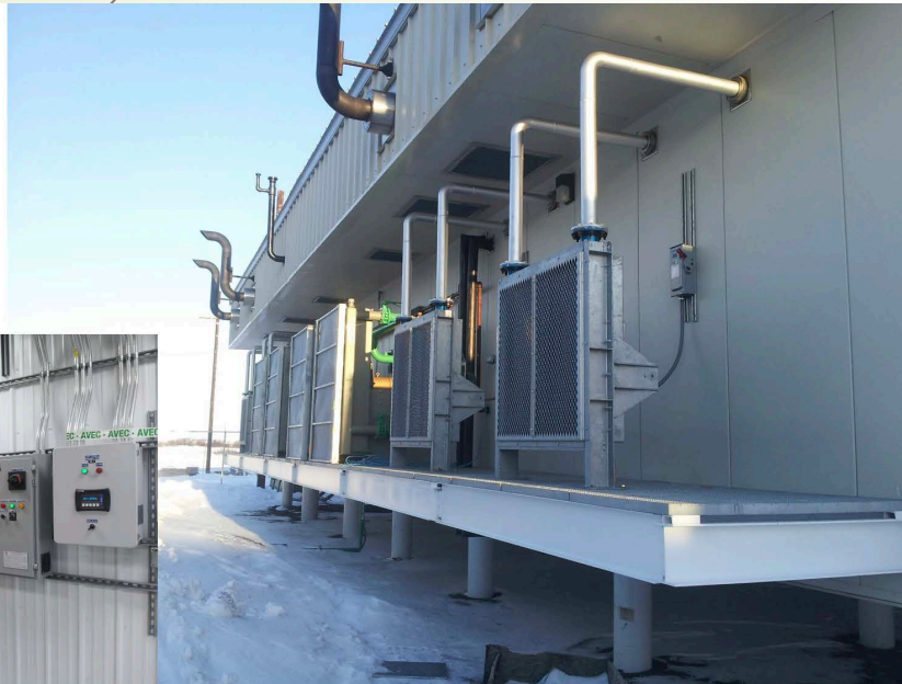
Remote Radiators with Variable speed Fans
