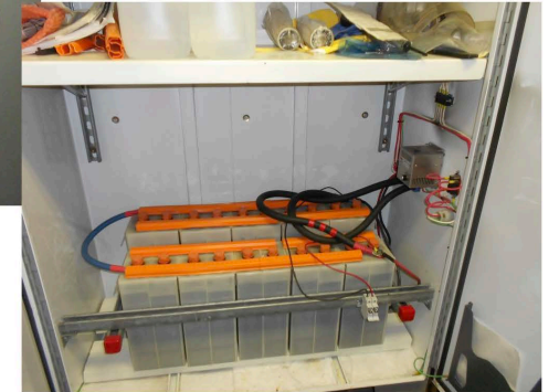
Nickle Cadmium Battery Bank
